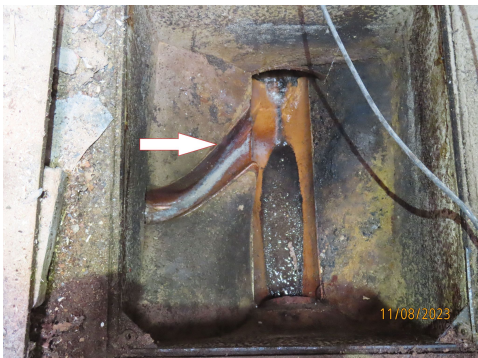
Front inspection chamber. Arrows indicate direction of flow.
