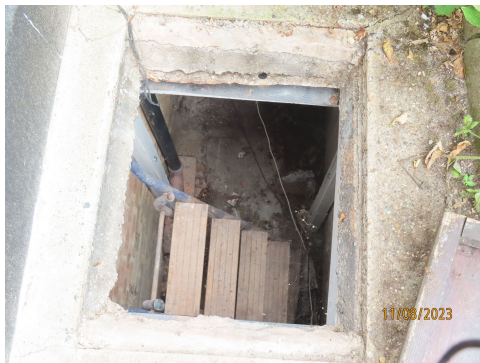
Access to basement
