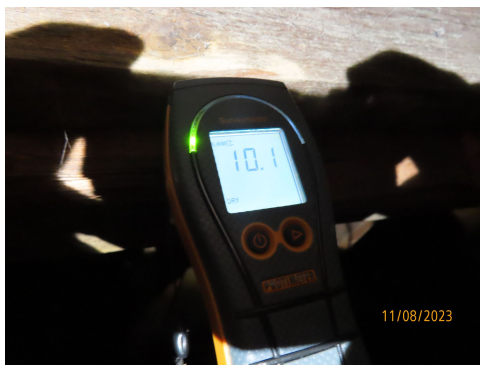
Moisture meter reading within normal range.
