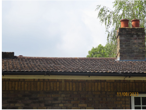
View of roof coverings
