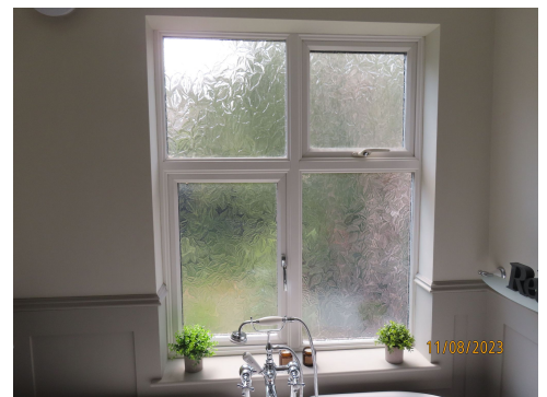
Low level window main bathroom
