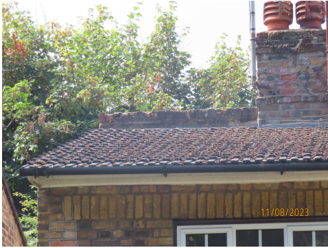
View of parapet section.
