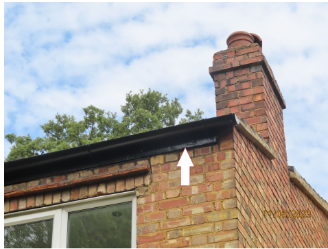
Timber fascia to rear
