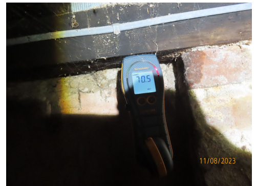
Timber moisture meter reading 70.5%
