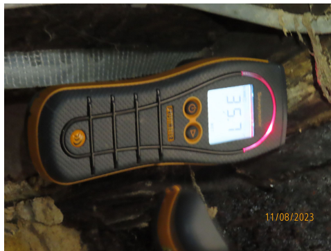
Timber moisture meter reading 35.7%
