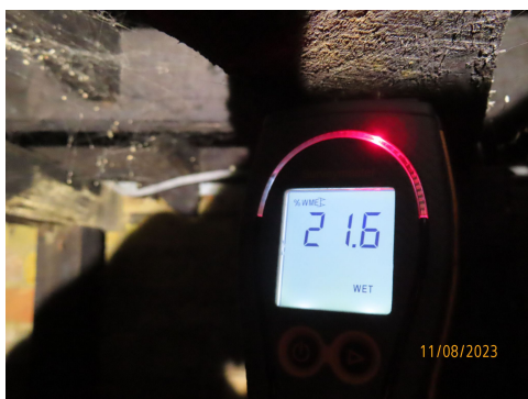
Timber moisture meter reading 21.6%
