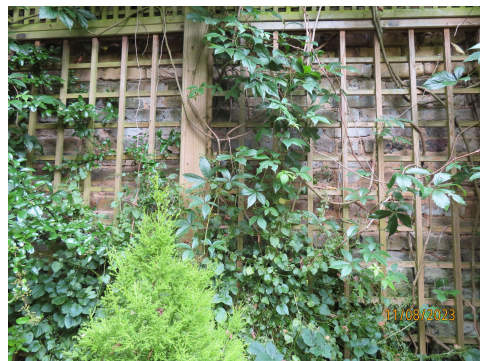
View of retaining wall to rear.
