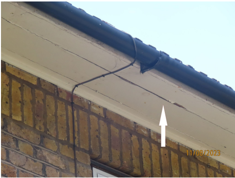
Timber soffit to front
